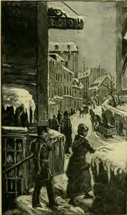
MOUNTAIN HILL, From top of Break-neck Stairs.
